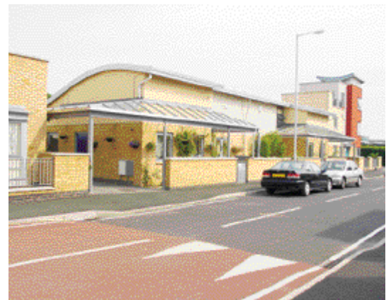
A range of different housing opportunities are well integrated to create a balanced community and a coherent street scene. Rolls Crescent, Hulme
