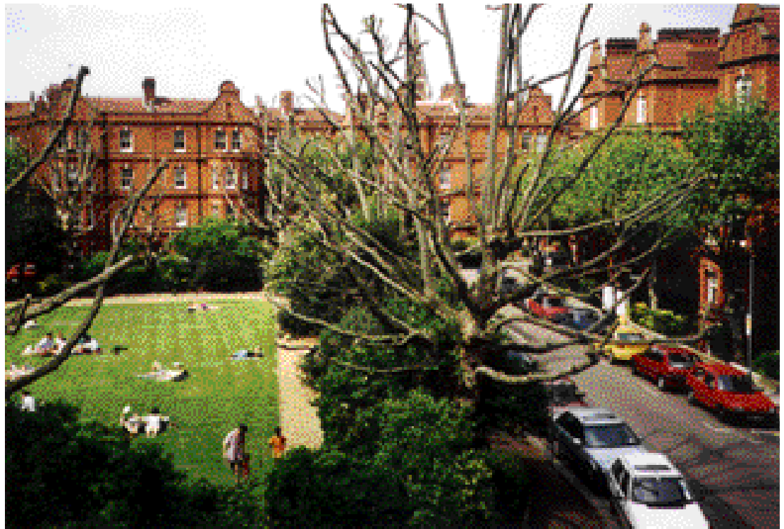
Urban apartments grouped around a shared green space. Here homes, landscape, routes for movement and parking are blended seamlessly together to create an attractive and distinctive place to live. Barons Court, Hammersmith and Fulham
