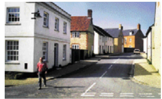
Tight corners and pinch points in the street encourage drivers to drive cautiously. Poundbury, Dorset
