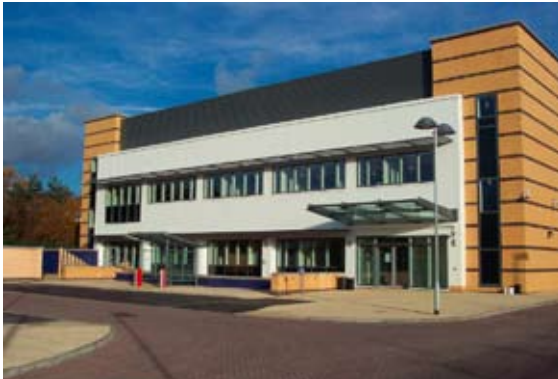
Figure 2 West Midlands regional control centre
