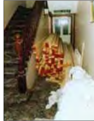
Figure 9: A blocked corridor with incorrect signage
